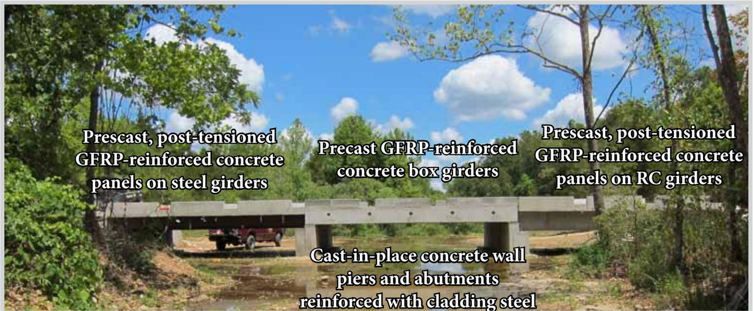
Figure 1. Complete three-span bridge over Arnault Branch, Washington County, MO
