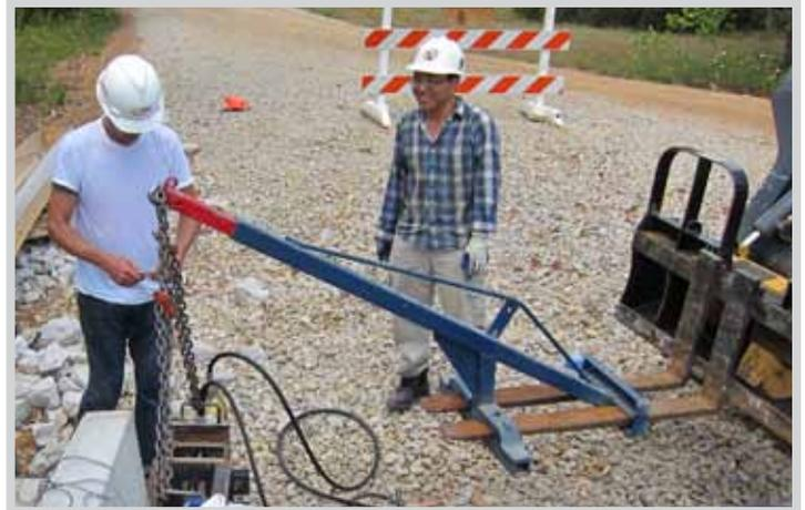
(b) Post tensioning of CFRP bars
