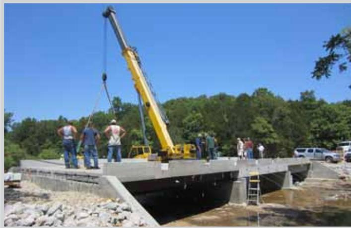
(a) Lift and placement of precast panel
